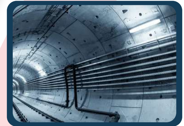
Feasibility Study of 500 kV Underground Cable 2×2000 MVA Transmission Line near Surabaya Airport
