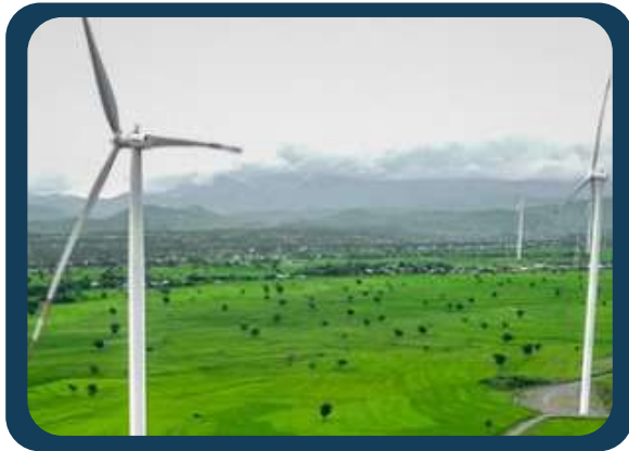
Tolo#1 Wind Farm Power Plant 72 MW Design Review , South Sulawesi, Indonesia
