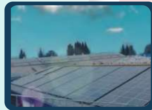
Structural & Roof Assessment at Danone Mekarsari Solar PV Rooftop Project West Java, Indonesia
