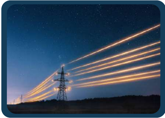
150 kV Transmission Line Preliminary Study for 250 MWp Solar PV Farm East Kalimantan, Indonesia
