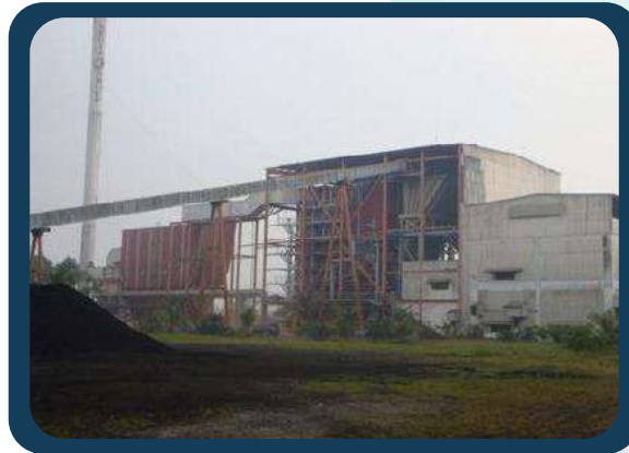
Operation and Technical Assessment of Coal Fired Steam Power Plant 15 MW (Aceh)
